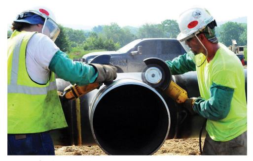
Fig. 3.3.3 Surface cleaning methods
