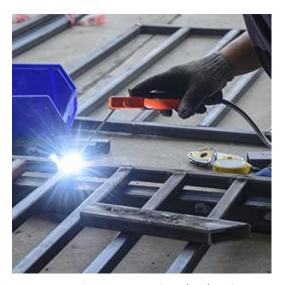
Fig. 4.3.14 Welding processes (MIG/TIG/Stick)
