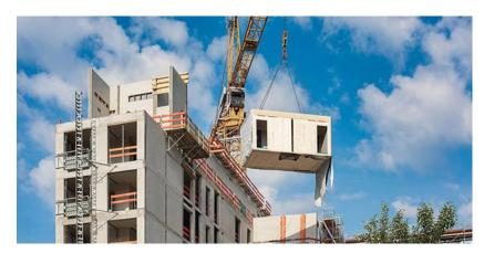
Fig. 1.2.3 Modular construction
