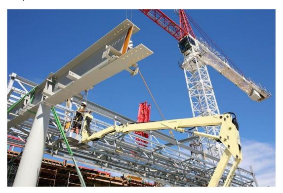
Fig. 5.2.5 Erection works in structural steel assembly
