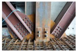
Fig. 5.2.2 Welding and permanent fastening
