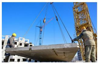
Fig. 1.1.17 Rigging work at site
