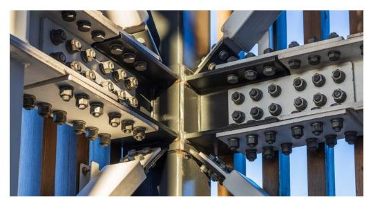
Fig. 5.3.5 Tightened bolted connection
