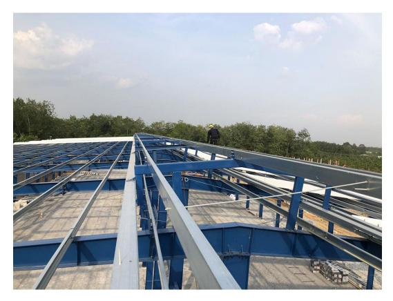
Fig. 5.2.9 Structural steel erections
