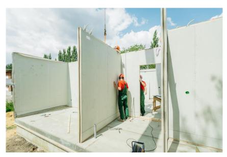
Fig. 1.2.2 Prefab wall panels
