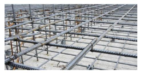
Fig. 1.1.12 Reinforcement bars fixed at site
