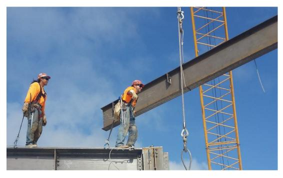
Fig. 5.2.1 Accurately placing steel components and making adjustments
