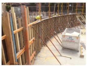
Fig. 1.1.13 Conventional formwork
