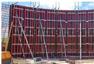
Fig. 1.1.14 System formwork
